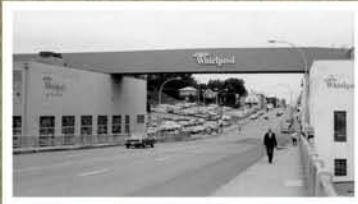
The Whirlpool plant straddled busy Arcade Street with a skyway used for moving production materials and finished products back and forth from the rail lines and loading docks to the factory buildings, ca. 1980.
