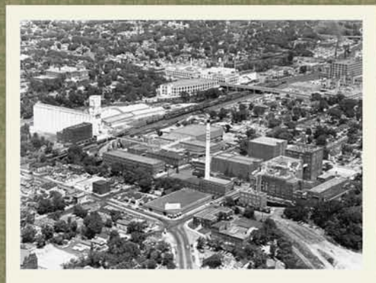
The last grain elevators and melting facility of the Hennin's Brewery once stood on this site. All around were leading industries and employers, including 3M, Whirlpool, and Northern Malleable Iron.
