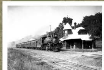
Railroads were important to the development of the Eastside, providing employment and affording the city's landscape. There was once a small commuter depot in the Highwood Hills neighborhood.
